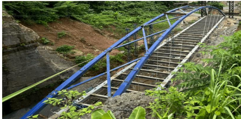
Fig. 15. Network arch steel framework fabricated at site
